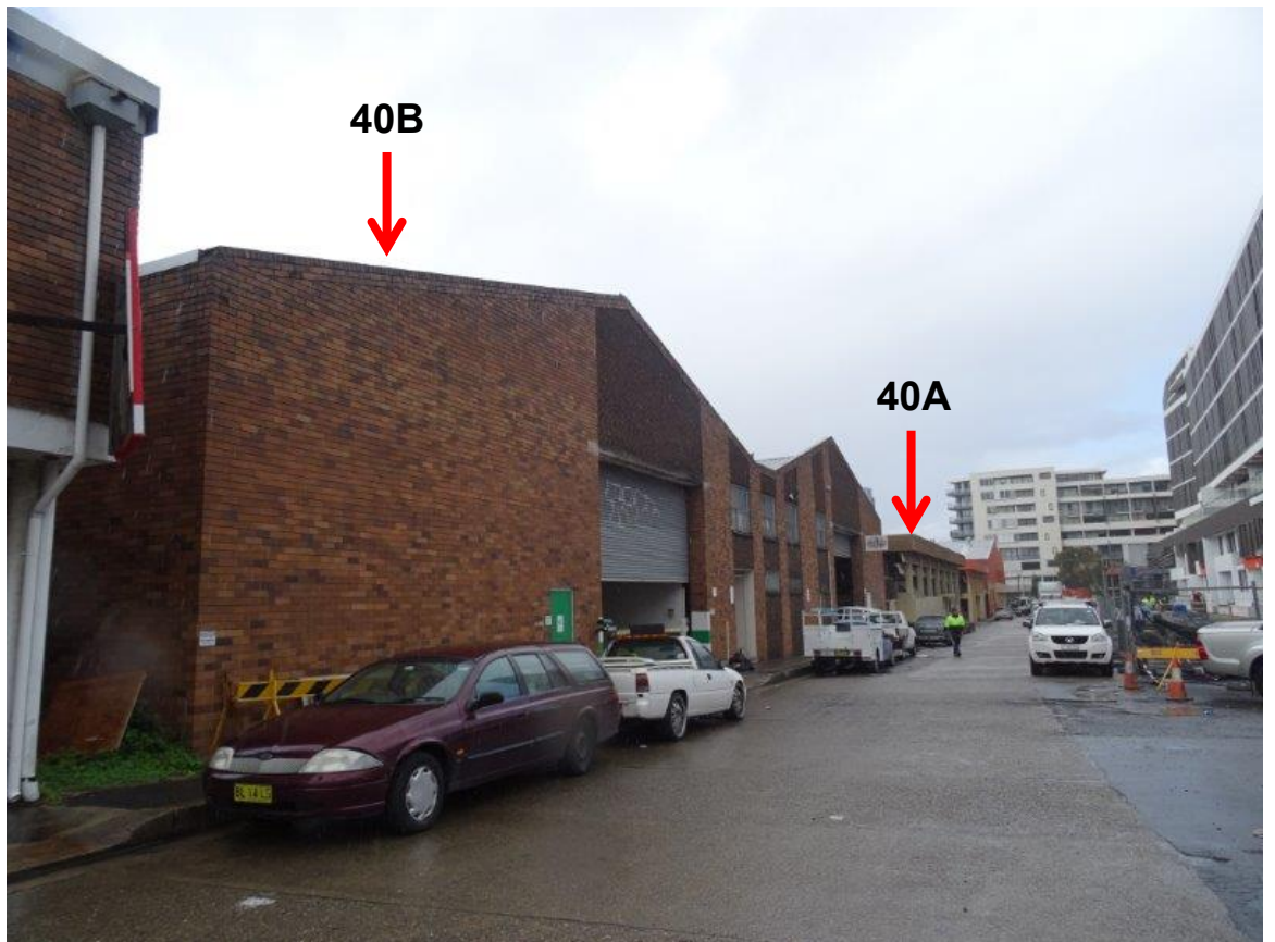
Figure 4: View of buildings on site, generally looking south down battle axe driveway.
